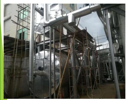
Compared to the original system, incorporation of PCM System, it is recorded that the daily electricity consumption is reduced by 882.98 kWhe (6150.2 - 5267.2) which correspondences to an energy reduction rate of approximately 14.36%
